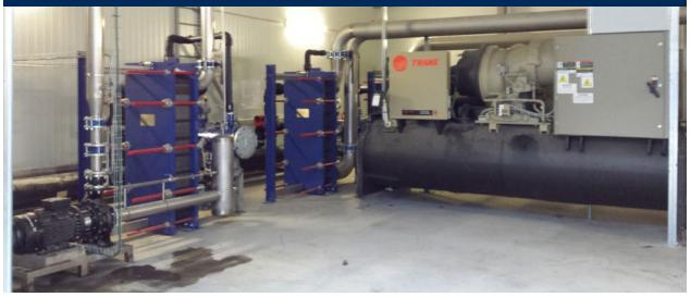
Exclusive system of refrigeration by sea water which was executed in the port and allowed to do without cooling towers and to reduce the energetic consumption of cooling equipments. A set of pumps installed in the seabed pump the water through a subterranean pipes system towards the services room where the water is returned to the seabed in a controlled temperature.
